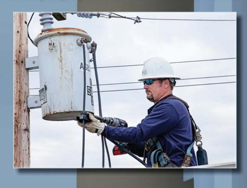
The SensorLink Transformer Meter provides utility groups with precise information to quickly identify inefficient Transformer loading due to power theft, without the requirement of Advance Metering Infrastructure.
