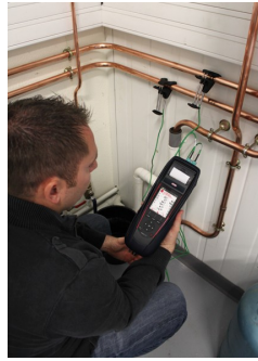
DHW network temperature
