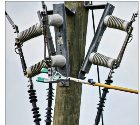
Standard Ampstik+ on Overhead Switch
